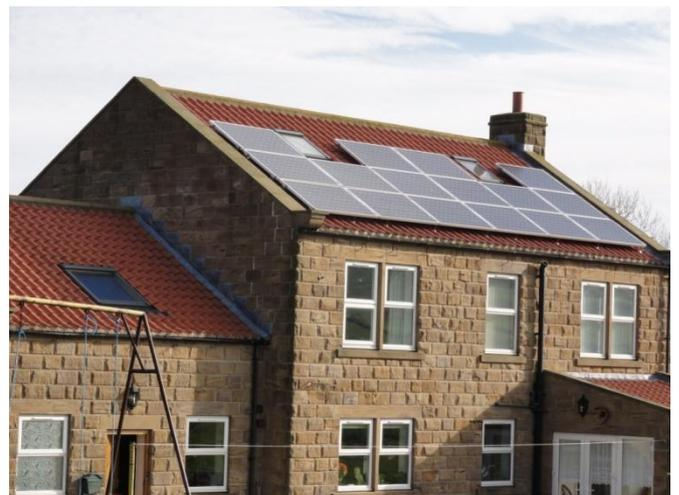
**Issues to consider:-** The system on the barn roof has two inverters, each for 8 panels. Any difference in output will indicate a likely fault. The inverter in the house is in a cupboard and a fault was not spotted for a while. A Bluetooth monitoring system is worth considering.
